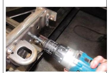
42. Replace the Ø13mm drill bit with a Ø10.5mm drill bit and pass the drill through the Ø13mm holes.
