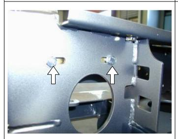
M8 bolts must fit in rear of bar for ease of adjustment later on.
