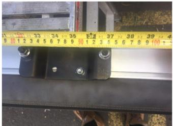
Install awning brackets on to awning and set at the required pitch taken from the previous step.
