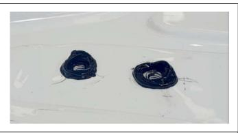
4. Spread a small amount of sealant around the anchor points.
